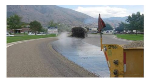
Chip sealing involves spraying an asphalt emulsion on the pavement, then immediately spreading a layer of uniformly sized aggregate chips. The new surface is rolled to seat the aggregate. After a twenty-four hour curing period excess chips will be swept up.
