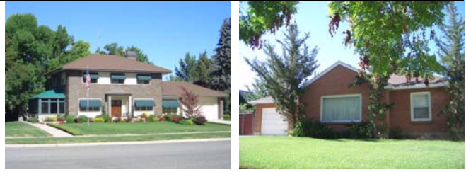
These attached front-loaded garages do not detract much from the houses, because they are recessed from the front planes of the houses and make up only a small portion of the front elevations.
