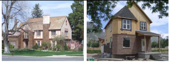
Left: the part of the second story that projects out past the plane of the brick wall has materials that appear light. Any other projections are supported directly by the foundation, allowing them to be constructed of heavy materials. Right: the brick bay that projects out from this new infill house should be supported by the foundation.
