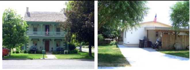
Left: appropriate elevation with sufficient wall space dedicated to windows and doors. The windows and doors are also balanced on the facade. Right: inappropriate front elevation with only two small windows, no entrance, and an imbalanced facade.
