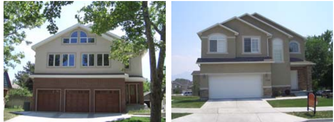
Both of these garages are inappropriate since they both are wider than 40 percent of the width of their houses. Neither garage is visually subordinate, since they both have prominent locations on the lot. Also, neither garage is set back from the front of the house; in fact the right one projects out from the front.
