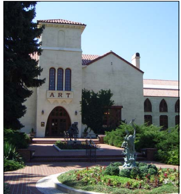
Figure 7-5 The Museum, built in 1937, is a Spanish Colonial Revival edifice located at 126 East 400 South
