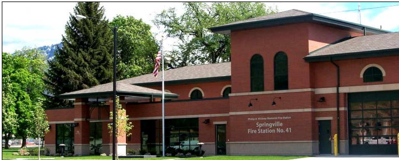
Figure 7-6 Fire Station built in 2009
