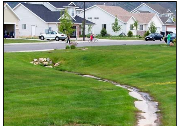
Figure 7-14 Camelot Detention Basin
