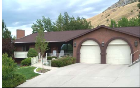
Figure 5-5 A single family residence typical of 1970-80s
