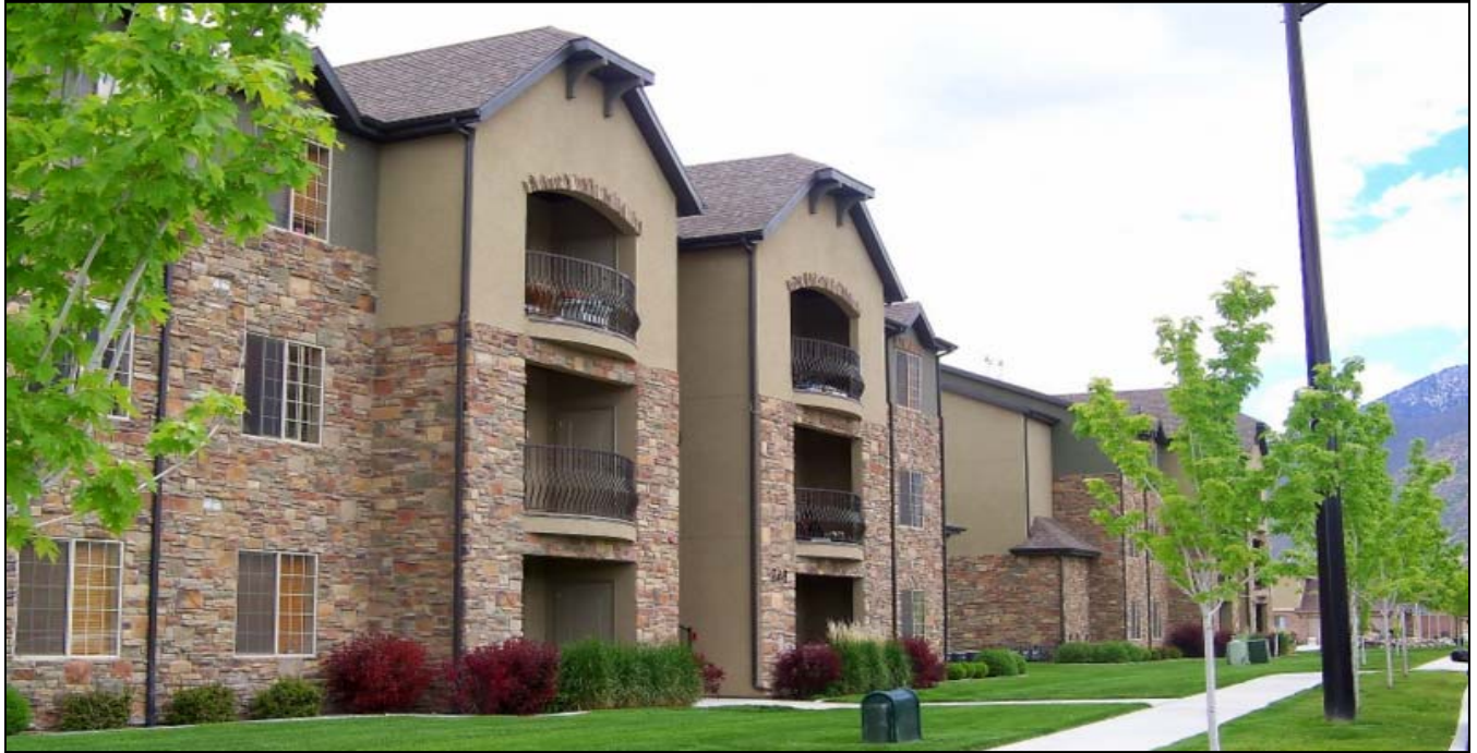
Figure 5-12 High density housing in Springville with a pleasant facade
