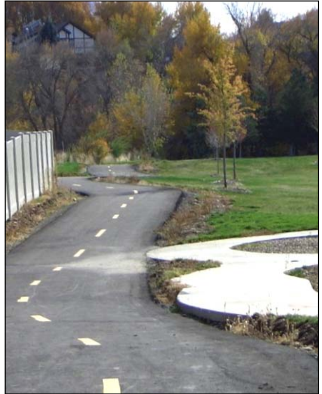
Figure 6-5 Portion of Hobble Creek Trail
