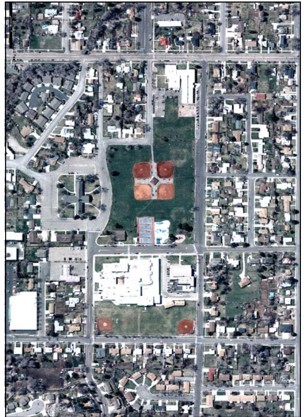
Figure 2-19 Located in the middle of the neighborhood, Memorial Park is surrounded by a church and elementary and junior high schools
