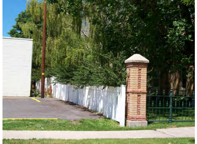
This photograph illustrates the parking area extending up to the edge of the commercial property.
