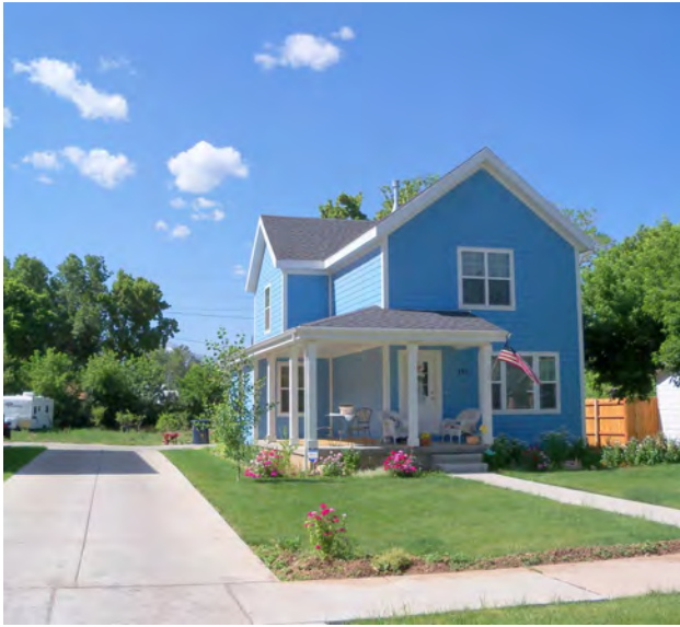
Figure 30 Historically appropriate infill construction.
