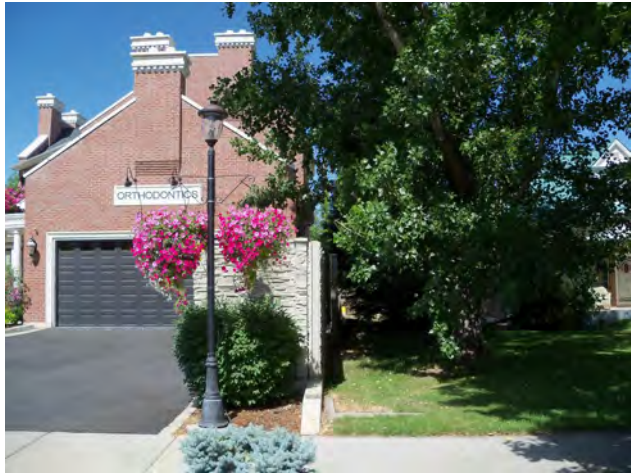
This illustrates an example of development before the ordinance was adopted, which allowed buildings set near the edge of the property without any transitional landscape buffer.
